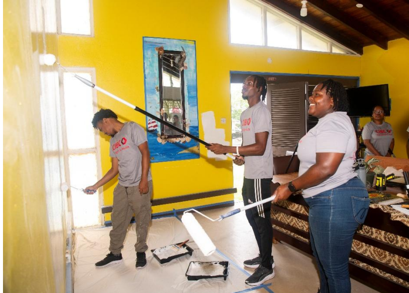
From left Tyrique Best, Aiden Alleyne and Sarah-anne Drakes all apply primer to the wall in preparation for repainting it.
