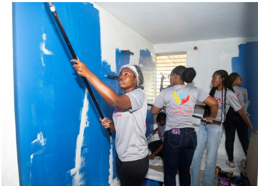
Niesha as she expertly applies the paint with the telescopic roller while the others work behind her.
